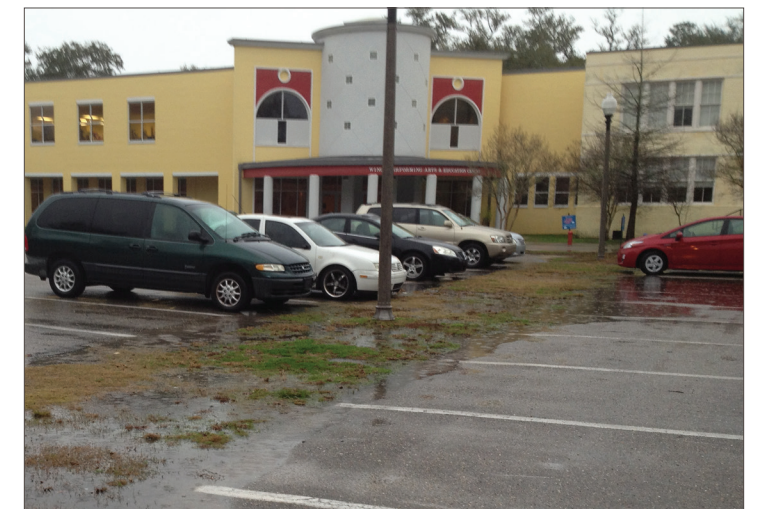
AESTHETIC & DRAINAGE ISSUES IN PARKING
