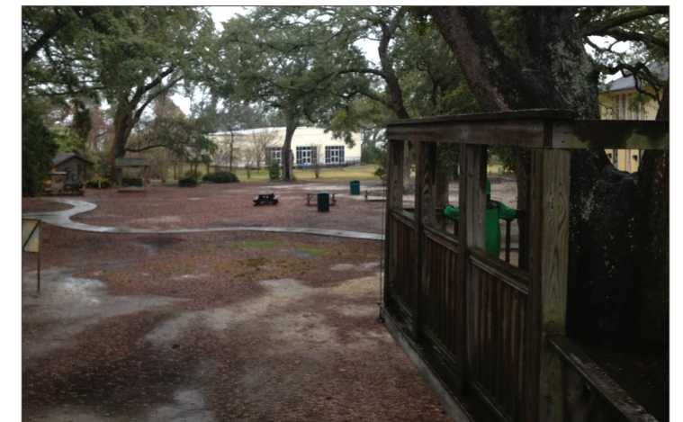
SURFACE & EROSION ISSUES
